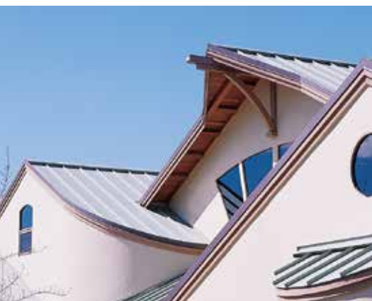
Factory notch allows panel to be field turned down with clean, uniform detail.
