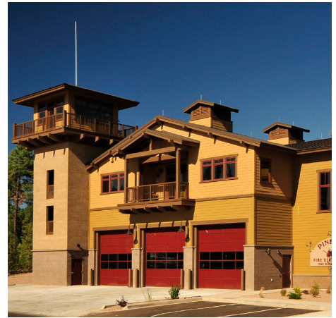
Pinetop Fire Station, Pinetop, AZ
